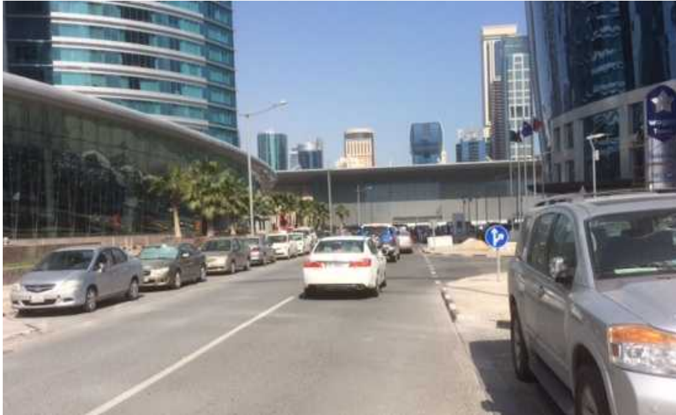
Figure 10-2: On-street parking through T-junctions is normal practice on the local streets throughout Qatar. Also evident is the nominal 6m setback from the tangent point to the start of parking on the right side of the street.
