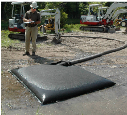
Figure 3.7 Gravity Bag Filter
